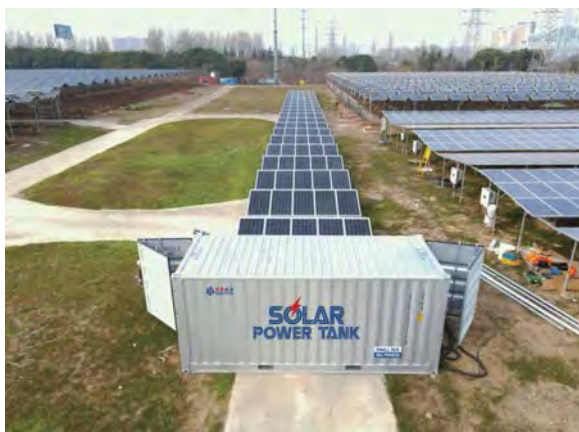
⑤ Cable Installation
