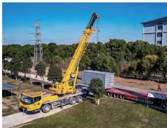
② Hoisting in Position
